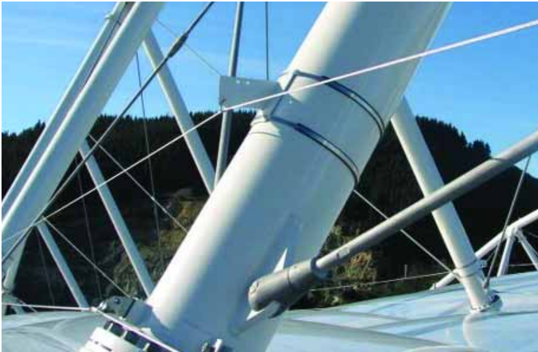
Jubilee clips fasten items of rigging to the main tubular structure
